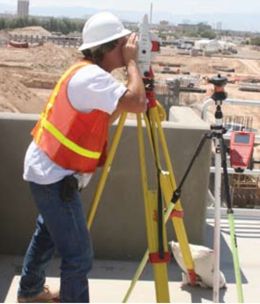
Simms takes a backsight with the Leica PowerTracker robotic total station.
