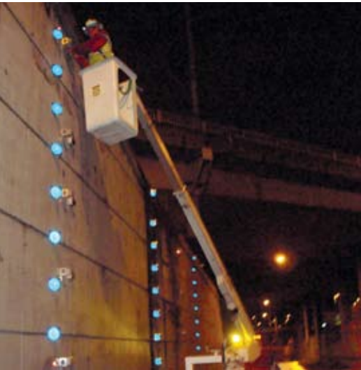
The laser scan targets were made of an aluminum base with circular laser scan reflective areas and a special horizontal angle offset to maintain perpendicularity to the laser scan locations.
