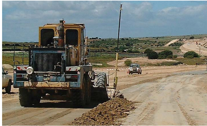
Leica System in use doing the final trim of stabilised material
