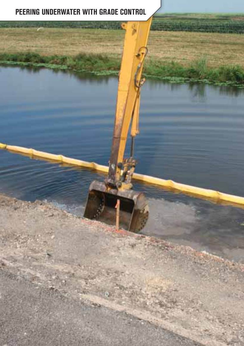
The slope of the canal bank is carefully controlled to prevent erosion.
