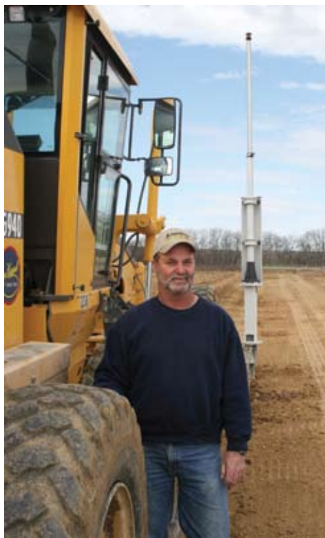
Bernie Schmidtlein recently lowered the cost of grading by making the move to automated grader control.
