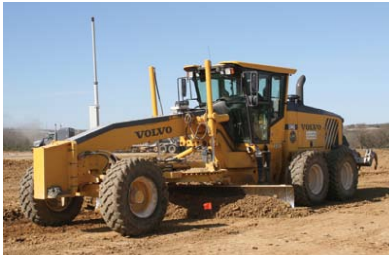
Schmidlein Excavating uses a Leica Power Grade 3D on a Volvo G940 motor grader.
