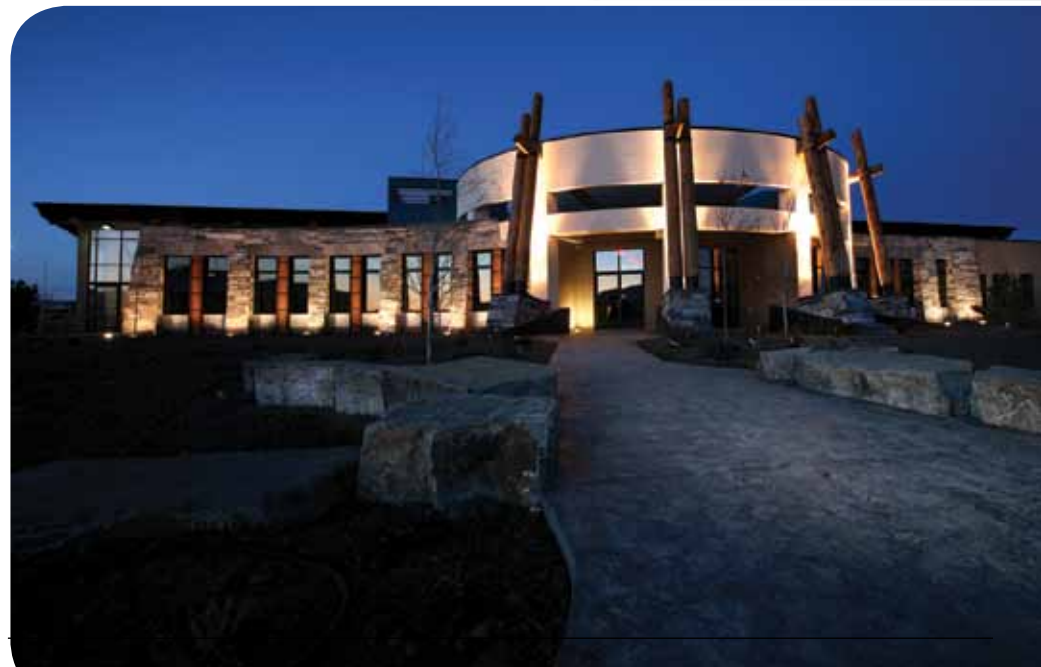
The columns are set at various spacings of typically 10 to 15 ft. apart. Note the curved radius wall, left, and the central atrium, right.
