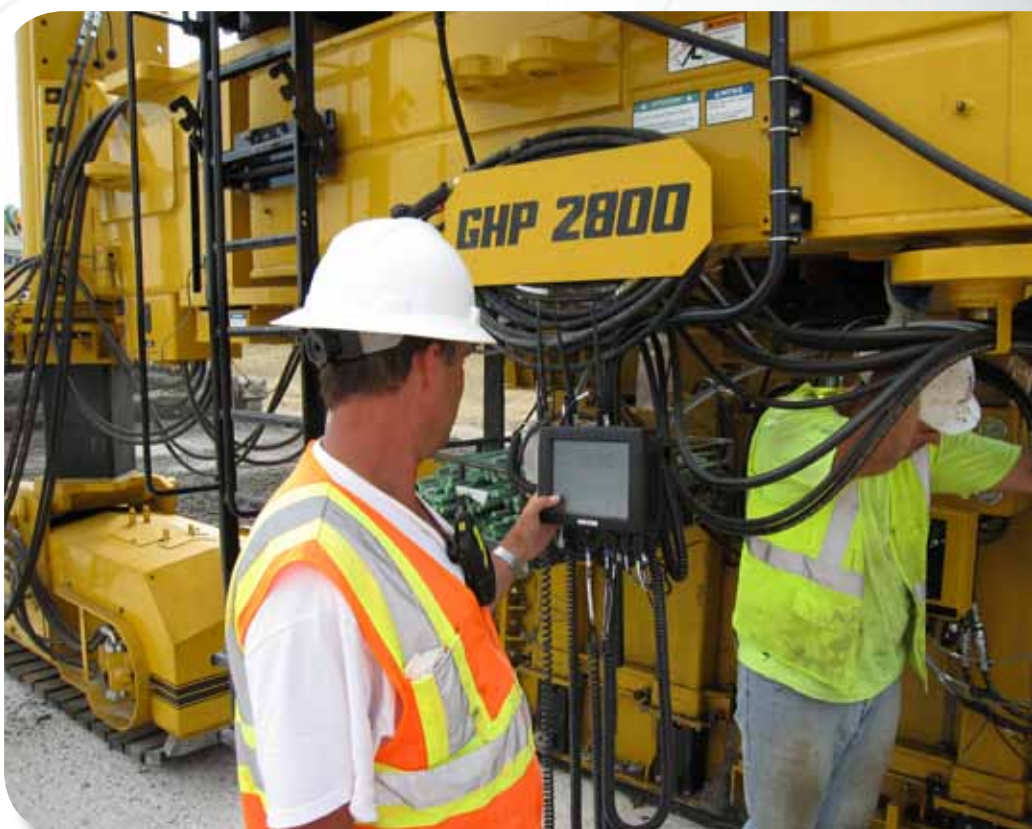
John VanMeter of Leica GeoSystems shows how the system is started on the GOMACO 2800 Paver.
